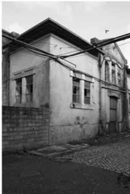
PHOTO | Existing Condition
