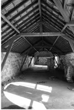
PHOTO | Existing Condition
